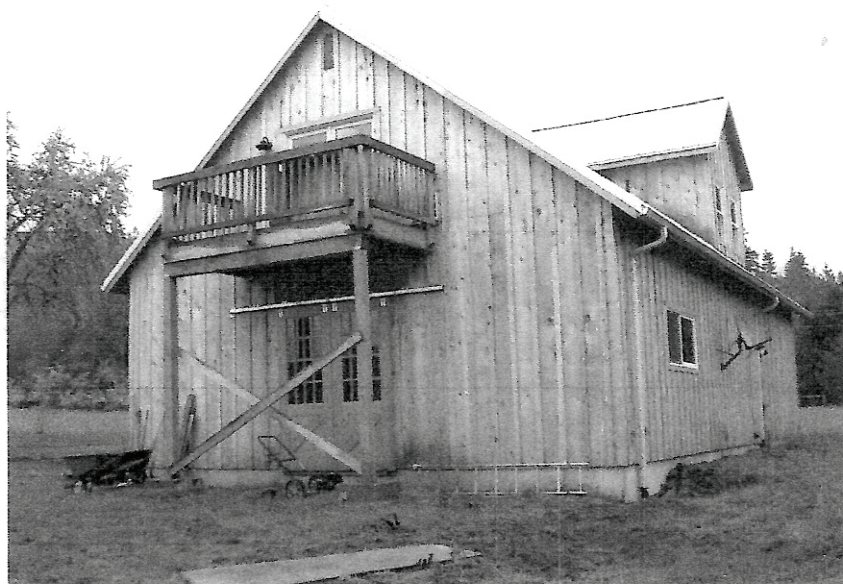
REAR (SW SIDE) OF CARRIAGE HOUSE. PHOTO TAKEN 04-01-09.
