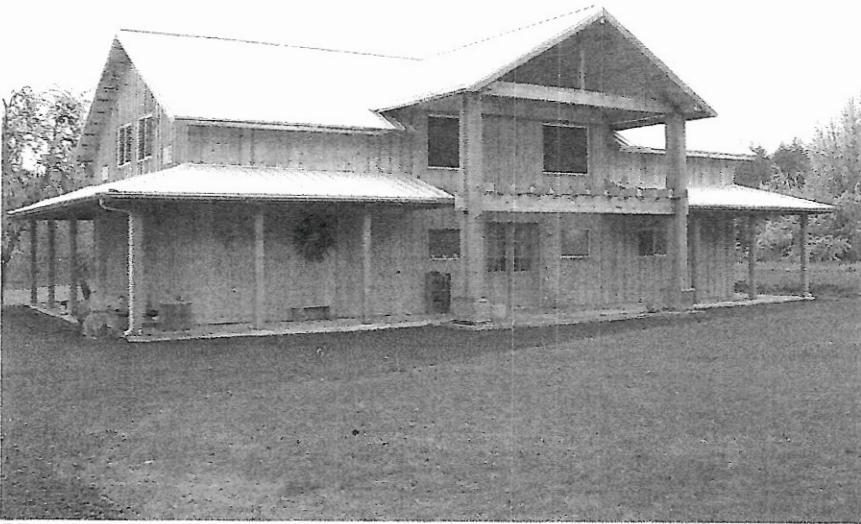
FRONT (EAST) SIDE OF MAIN HOUSE. PHOTO TAKEN 04-01-09
