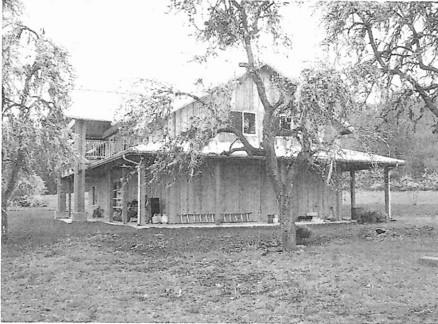
REAR (SW SIDE) OF MAIN HOUSE. PHOTE TAKEN 04-01-09.
